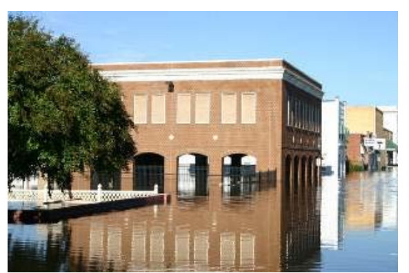
Downtown Franklin during the October, 2006 flood. Source: City of Franklin photo
