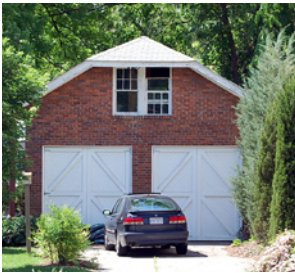
Keep and maintain historic features of a garage, such as windows and doors.
