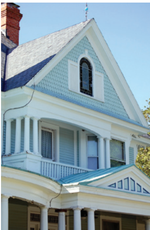
Exterior materials help express architectural style. The wood shingles, weatherboard, cornerboards, and window molding all contribute to the surface texture of this Queen Anne house.
