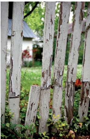
Replacing missing pickets eliminates weak points in a fence. Keeping pickets painted protects the wood from rot.
